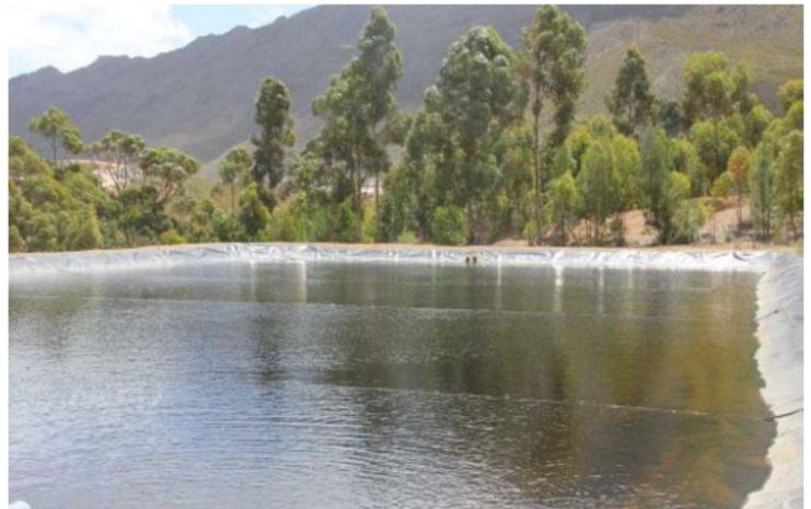
3 Ml Storage dam for supply from Kommissiekraal, Elandskloof and boreholes
